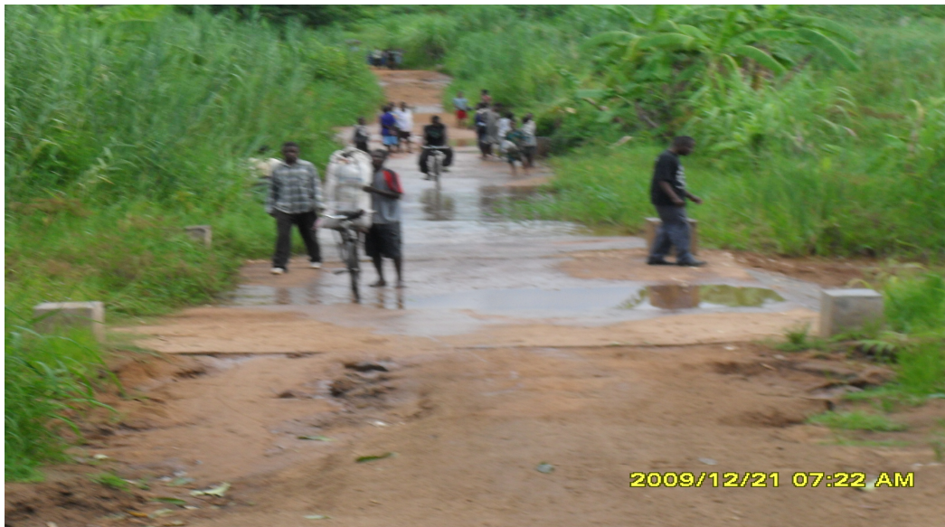
Figure 1 Figure 2.1: State of the road to village from Chingale turn-off
